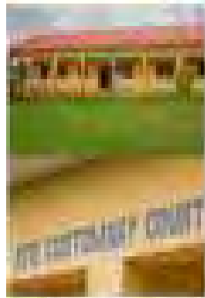
Complete renovation and rehabilitation of the Customary Court
